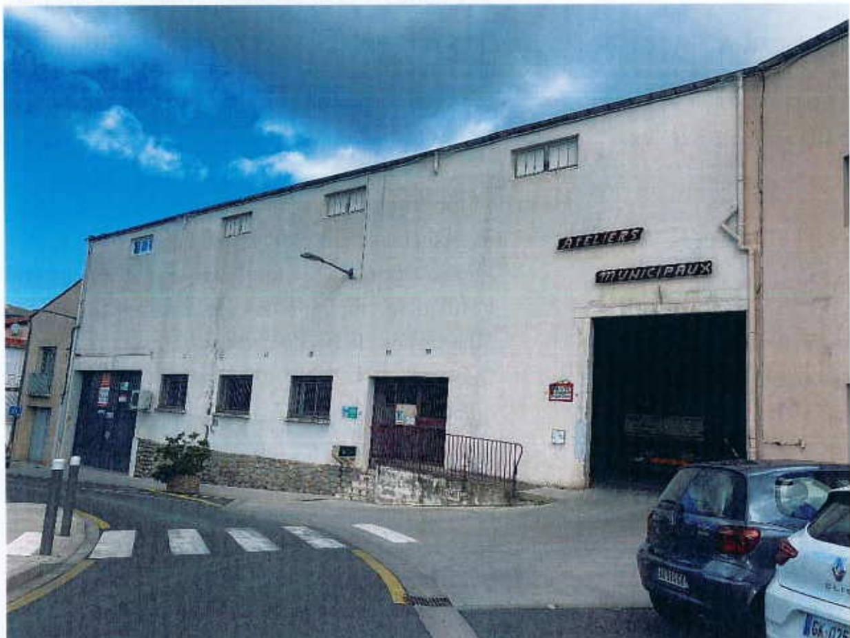
Figure 9 : Le centre technique municipal
